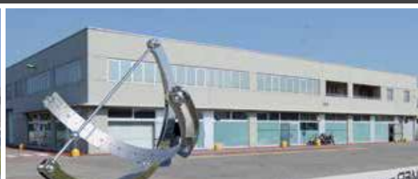
REMER ENGINEERING 1 high-tech production, R&D.
